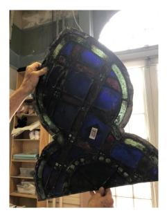
Above: Deteriorated pieces of the Rose Window with dirt accumulation, bowed glass, and cracked joints; the glass is cleaned, putty removed and replaced under each lead joint, and each piece re-flattened...
